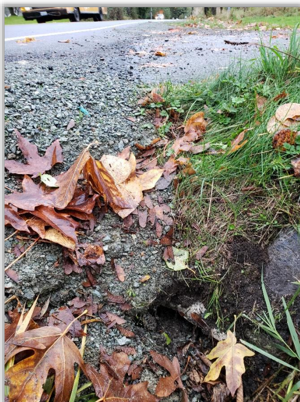
Photo S4, left: Looking south, a buried culvert of unidentified material conveys runoff in ditch under second driveway. Photo taken approximately 532 feet downstream.
