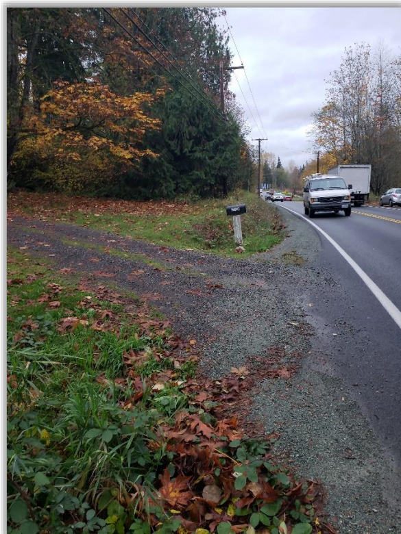
Photo S3, left: Looking north, ditch continues southerly and flow through 12" concrete culvert shown in Photo #2 and daylight 22 LF south, 82 feet from site.
