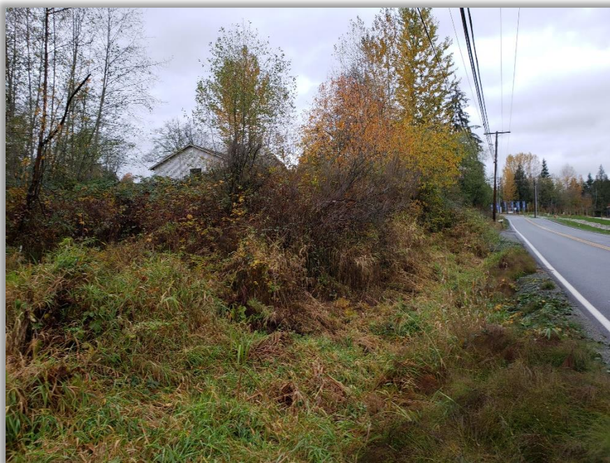
Photo N1, left: Looking north, sheet flow from site's north basin flows easterly to ditch along west frontage of Chain Lake Road right-of-way and converges to a single natural discharge point as shown in photo.
