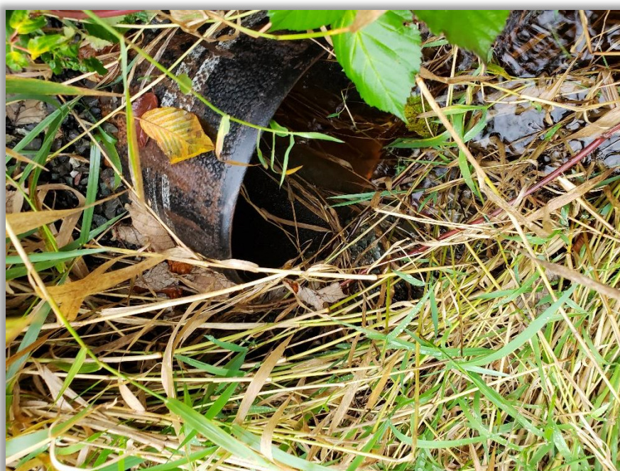
Photo N2, below: Looking southerly, a close-up photo of a 12" PVC pipe culvert in great condition conveys runoff 44 LF southeasterly where runoff daylights into vegetated stream.
